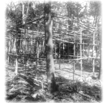
Site of the new church
